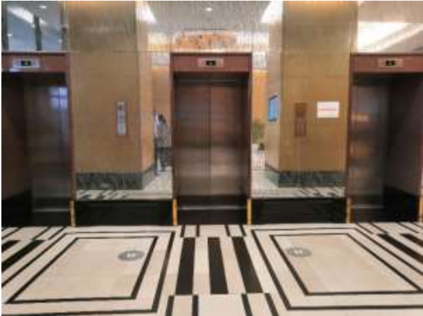
QUARANTINE: 2 elevators are designated (G2 and G3)
